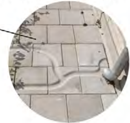
Waterplossing in de bestrating
