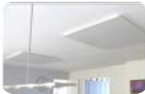
Infraroodpanelen
